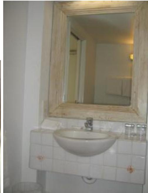
Clearance to the under side of the sink is 640mm with a height to top of sink at 760mm. The base of the mirror from floor is 1030mm.
