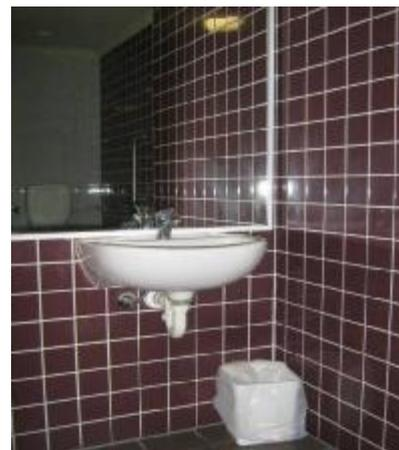
Clearance to the under side of the sink is 645mm with a top height of 800mm. The base of the mirror from floor is 830mm.
