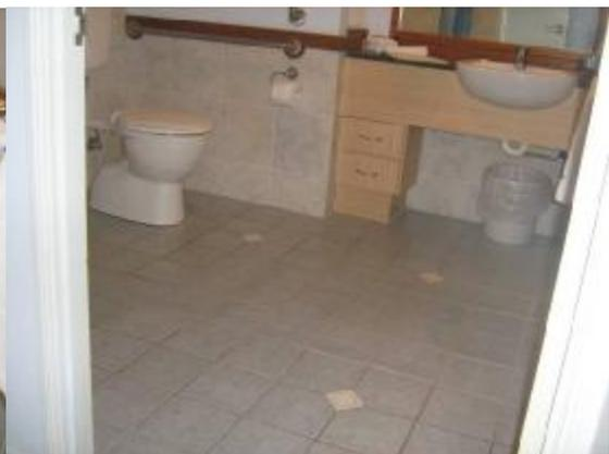
Clearance to the under side of the sink is 670mm with a top height of 810mm. The base of the mirror from floor is 880mm.
